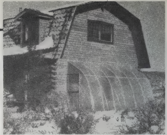
The Solar Room.
